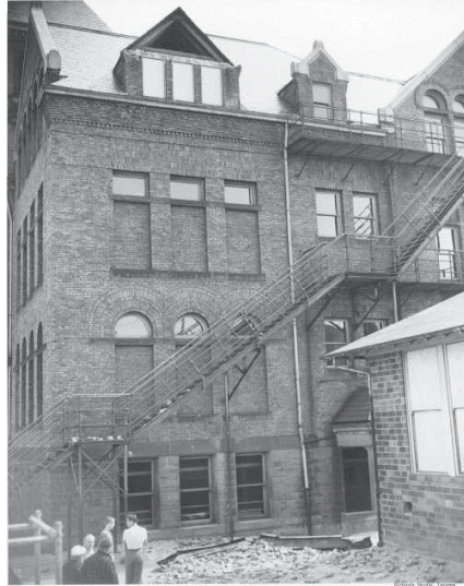
(TPL photo) In foreground - fallen bricks which covered boys
